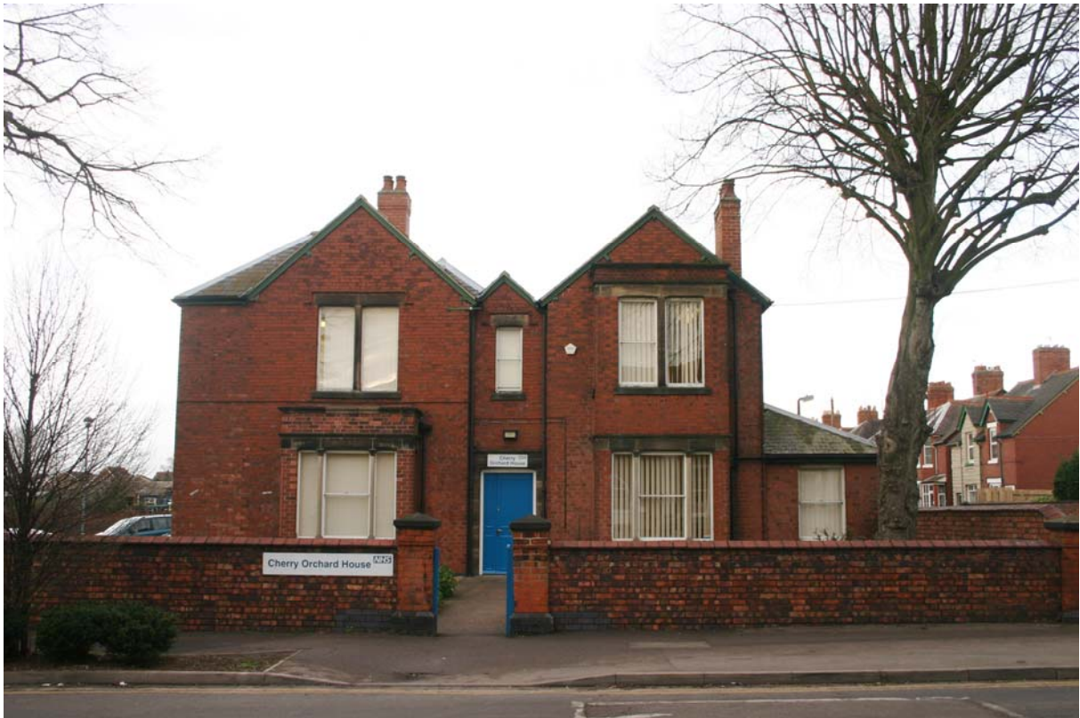
The locally listed Cherry Orchard House has been altered but still makes a contribution to the conservation area
