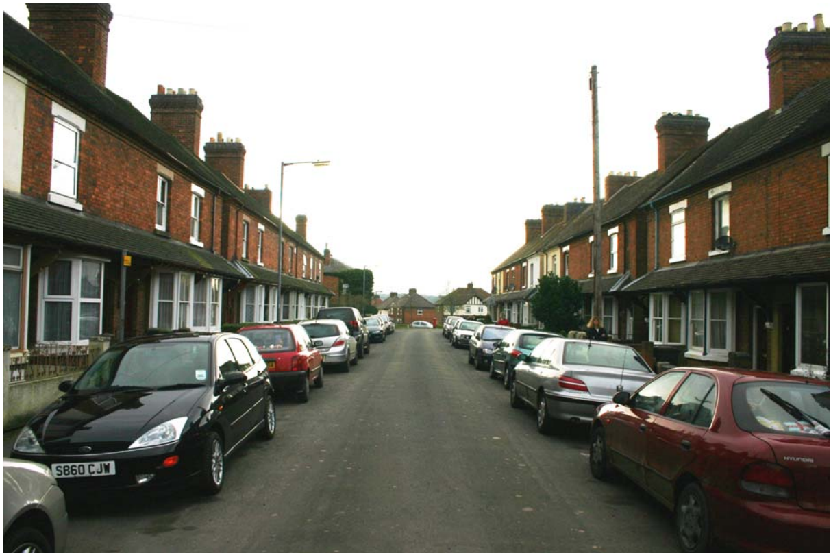
View west along Barbara Street; the continuous 'lean-to' roofs over the ground floor, the prominent chimneys, and the canted bay windows create a visually unified streetscape
