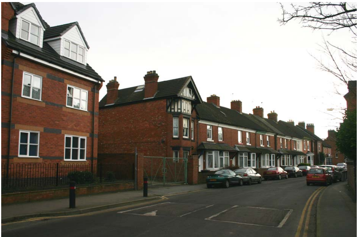
The gentle curve in Hospital Street drawing the visitor on into Barbara Street, No.29 is visually important in the street scene due to its height
