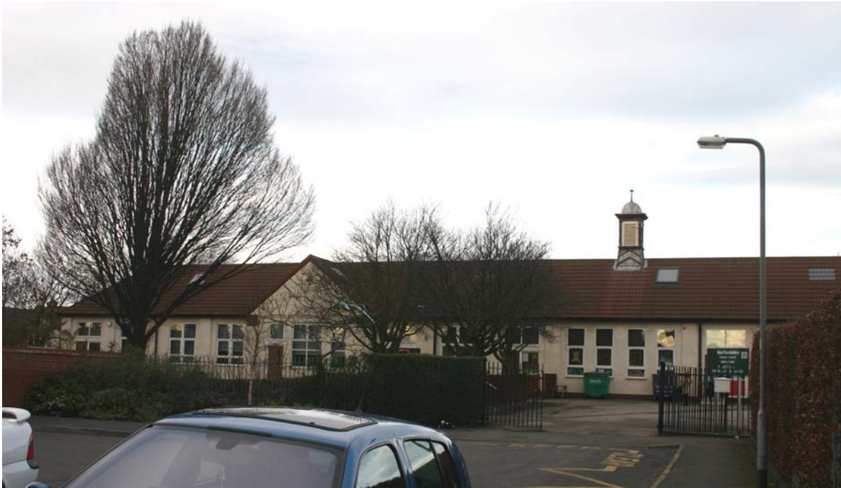
Primary school building (much altered) at the northern end of Moorgate
