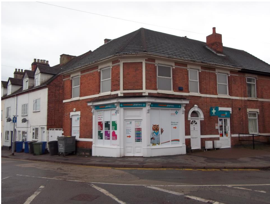
Figure 1 – Inappropriate signage at 54-54A Albert Road.
