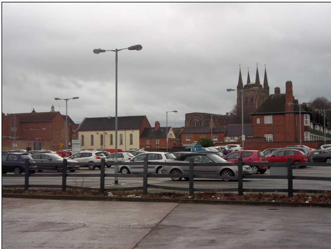
Figure 2 Surface Car parks impact negatively on the character and appearance of the Conservation Area
