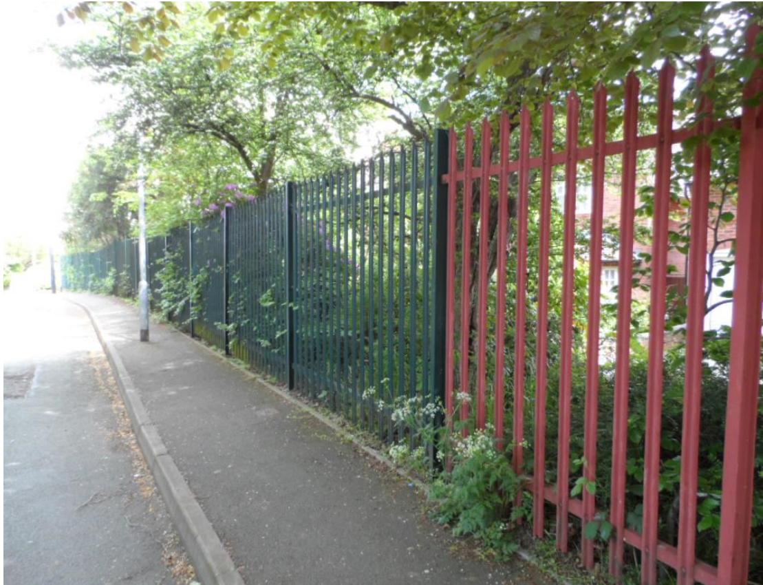
Figure 2 – Palisade Fence, Glascote Lane.
